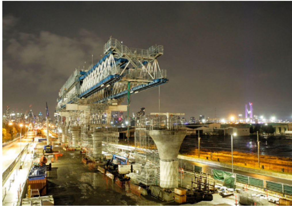
Capacity: 120 t/1280 t Span: 45 m AUSTRALIA Span by span erection
