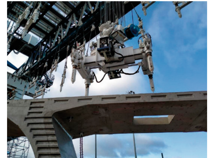
Automatic hanging system for span erection
