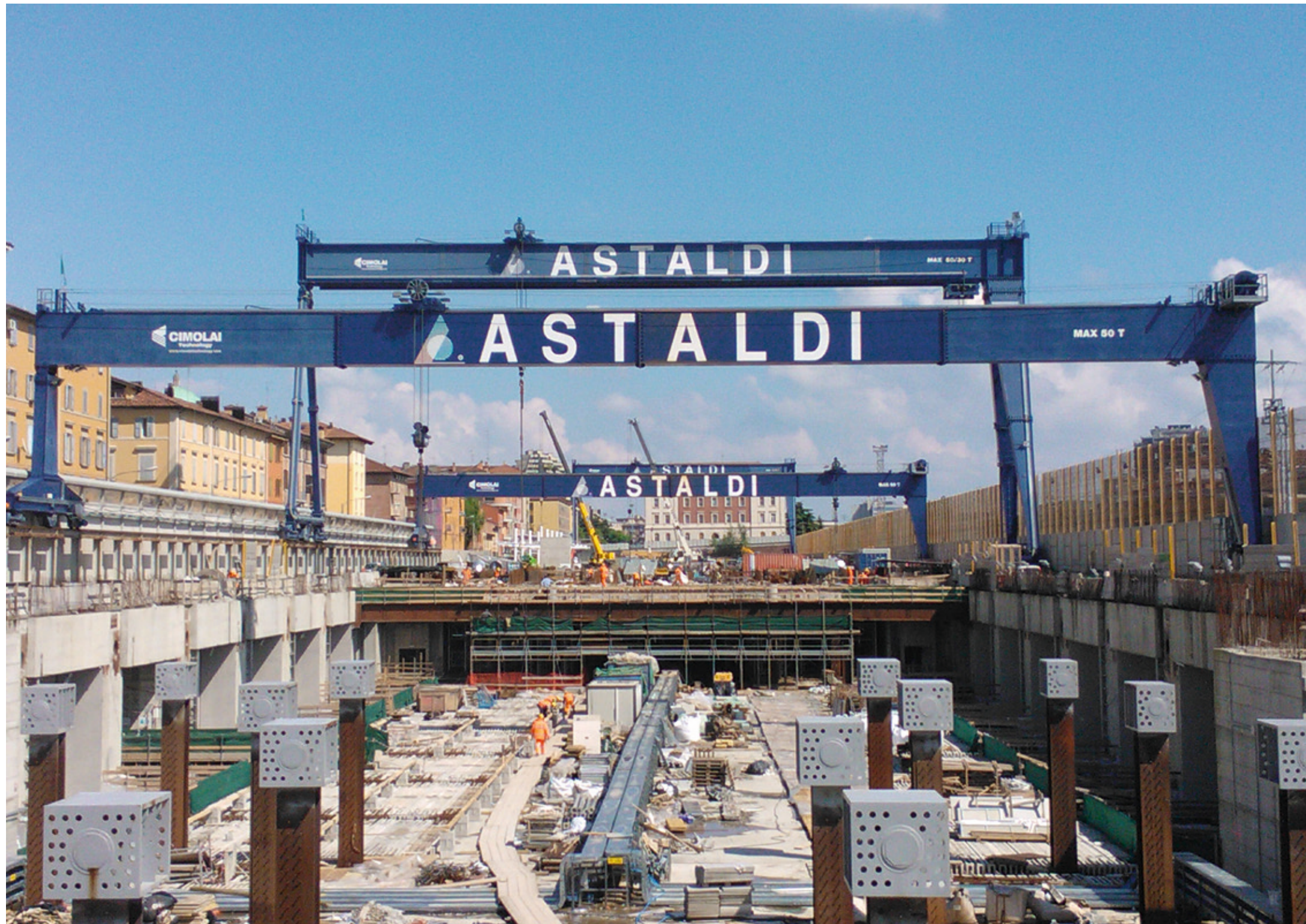
Capacity: 100 and 50 t Span: 57 m ITALY Gantry crane for the construction of underground station
