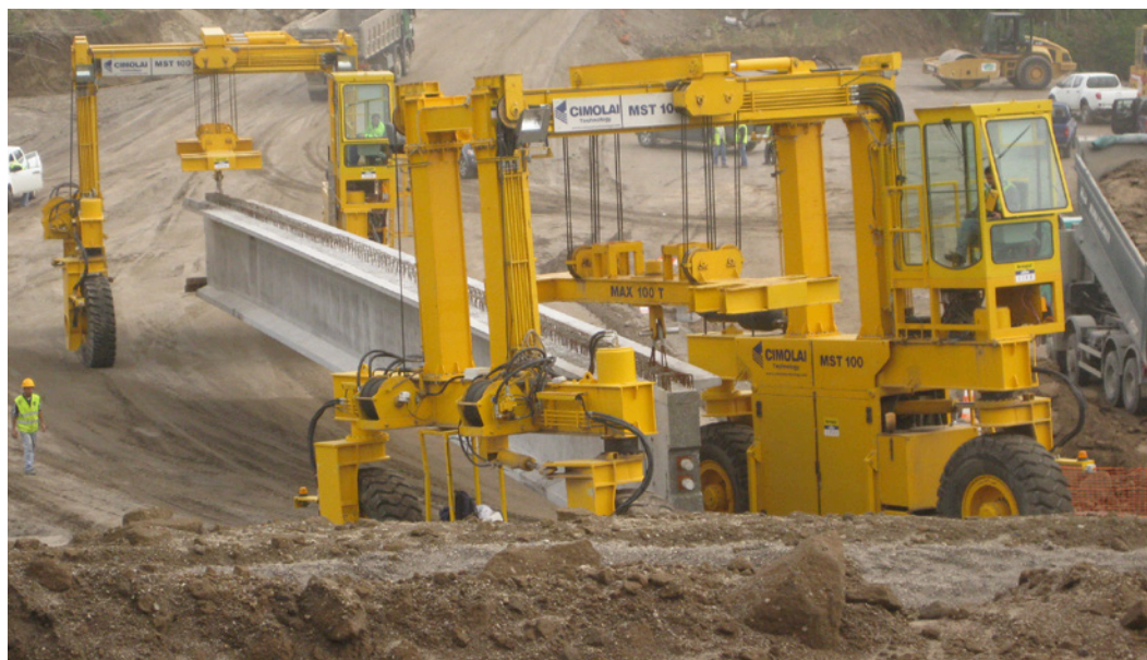
Capacity: 100 t /each SPAIN N.2 units suitable to be used in tandem
